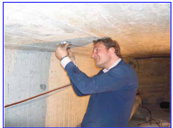
Figure 13b: Mounting of a fiber-optical strain sensors on the roof of the girder box. The fiber-optic string covers 5 m on each side of pylon 2.
