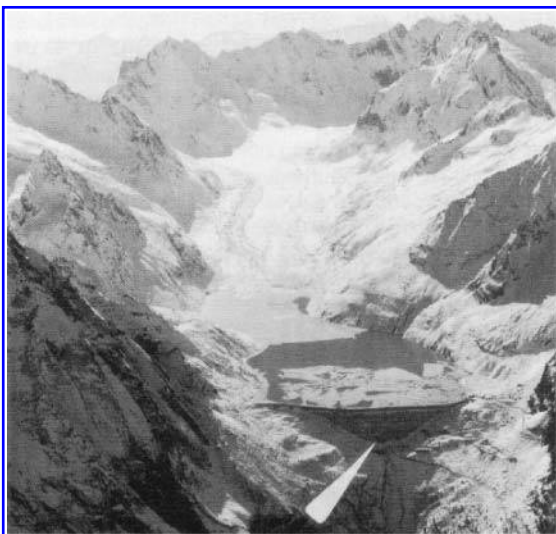
Figure 5a: The Albigna dam, which has considerable alluvial deposits in its immediate reservoir area, deforming the dam foundation on impoundment.
