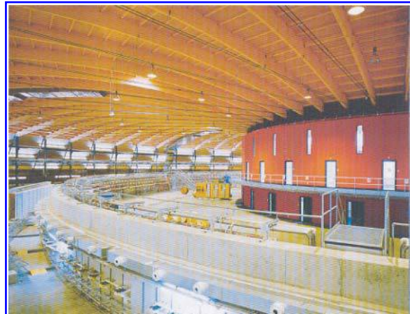
Figure 8b: Storage ring of the SLS during construction.
