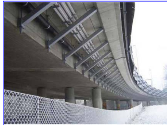
Figure 11b: Enlarged part of the bridge, bottom view.
