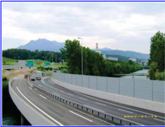
Figure 11a: Highway bridge near Lucerne after enlarging during construction phase, top view.
