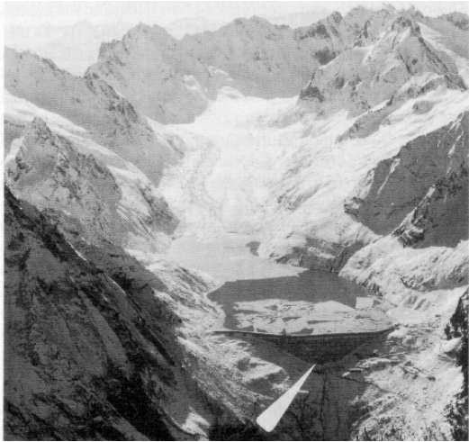
Fig.6 - The Albiga reservoir in the Bergell valley, Switzerland. An arrow marks the place where the hydrostatic measuring system is mounted in the dam. The dam has the direction East-West with the reservoir in the South.
