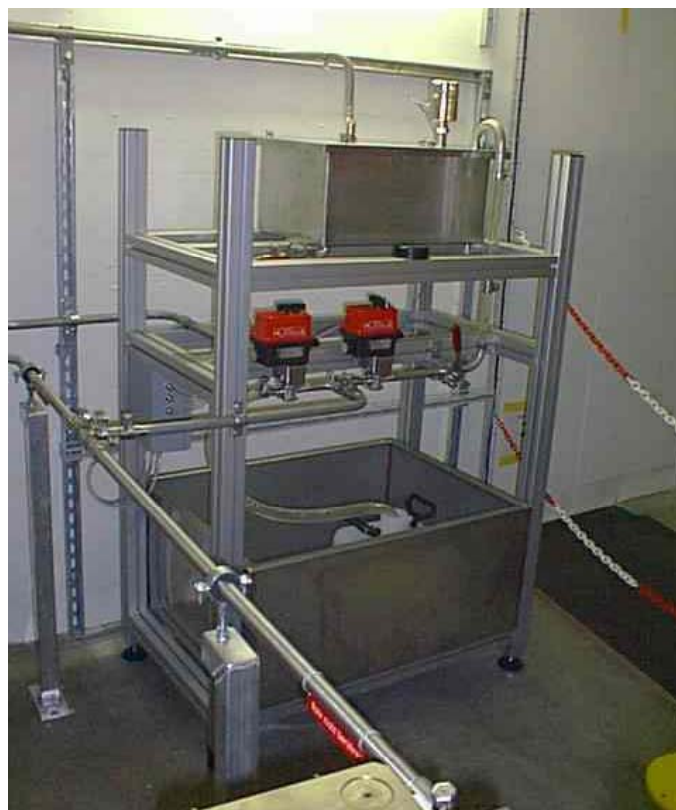
Fig. 8: Inner filling station. The two red pumps for draining (left) and refilling (right) of the HLS can be completely remote controlled. The inner filling station is directly connected to the half-filled HLS pipes which can be seen at the lower left corner of this figure.
